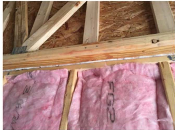
An example of foam applied at the seam of top plates.
