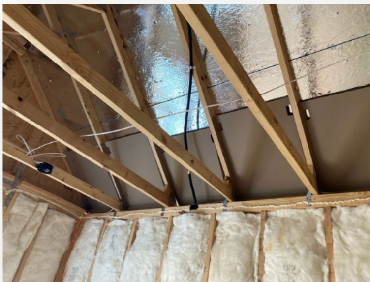
Figure 2 Thermal barrier roof board. The underside of this sheathing has a layer of reflective foil.
