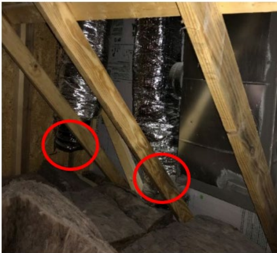
Figure 3 Examples of unconnected ducts in the attic and garage space at rough inspection
