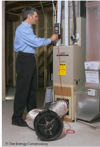
Figure 1 Duct blaster test set-up and connected to furnace
