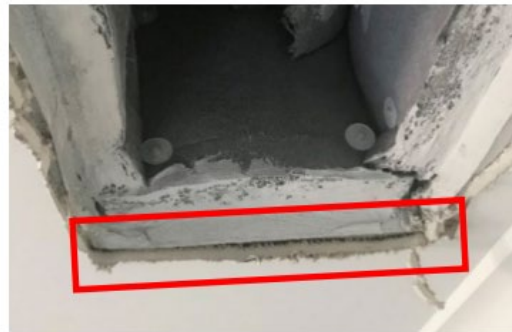
Figure 2 Examples of an unsealed supply and return
