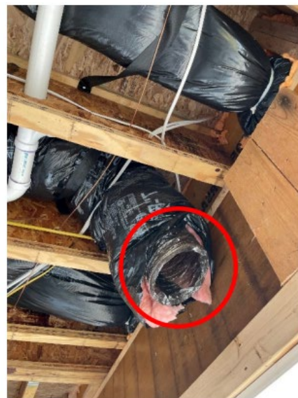
Figure 3 Examples of unconnected ducts in the attic and garage space at rough inspection
